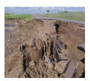
In June 2010, outflows from Maple Creek exceeded the capacity of two existing culverts under Highway No. I. Water overtopped Highway No. I, washing out 100 m of the westbound lanes and damaging 200 m of the eastbound lanes, leaving an 11 m high crater.
